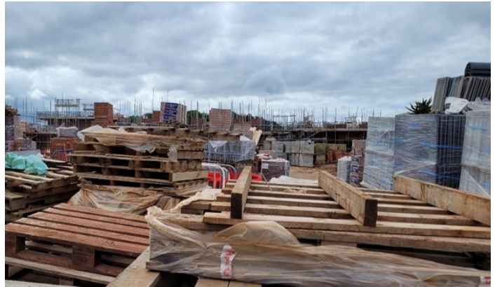
Dwellings under construction beyond Musters Road
